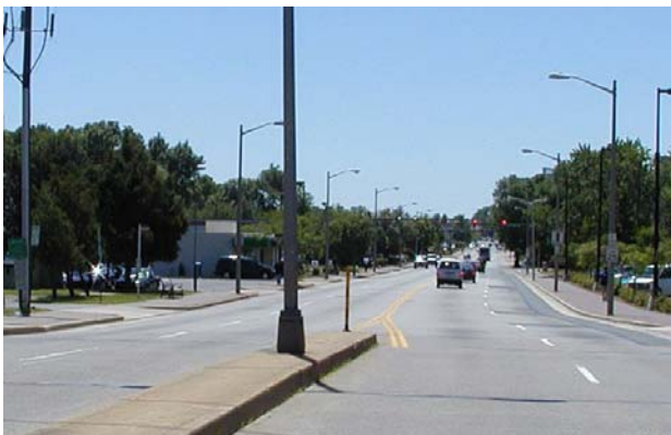
Existing condition looking south
